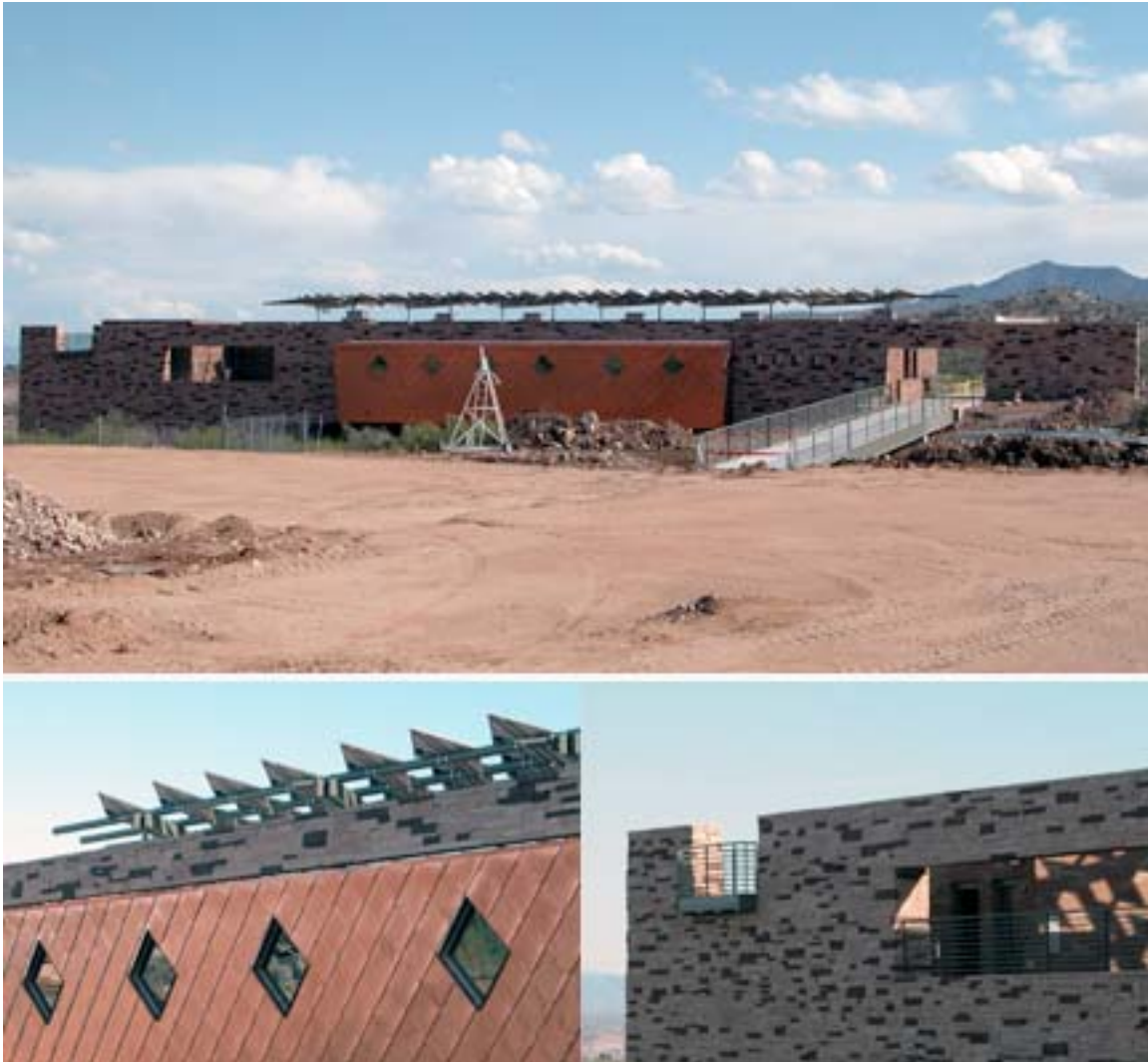
Figure 15: Views from NW show the photovoltaic shading structure hovering over the building, with patterns of light and shade appearing on the patio walls.
